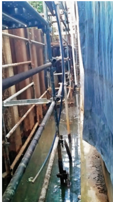
The application where the pump was operating to remove seepage water
