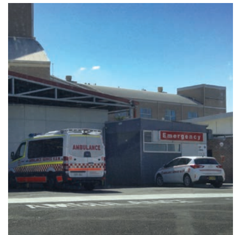
EMERGENCY DEPARTMENT WHERE HOT WARM WATER IS CIRCULATED
