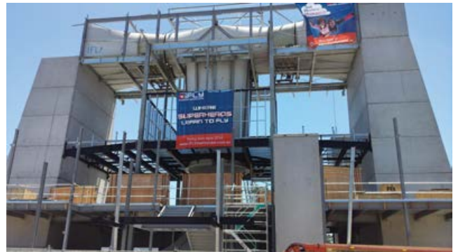
Australia's first indoor skydiving centre during construction in Penrith NSW
